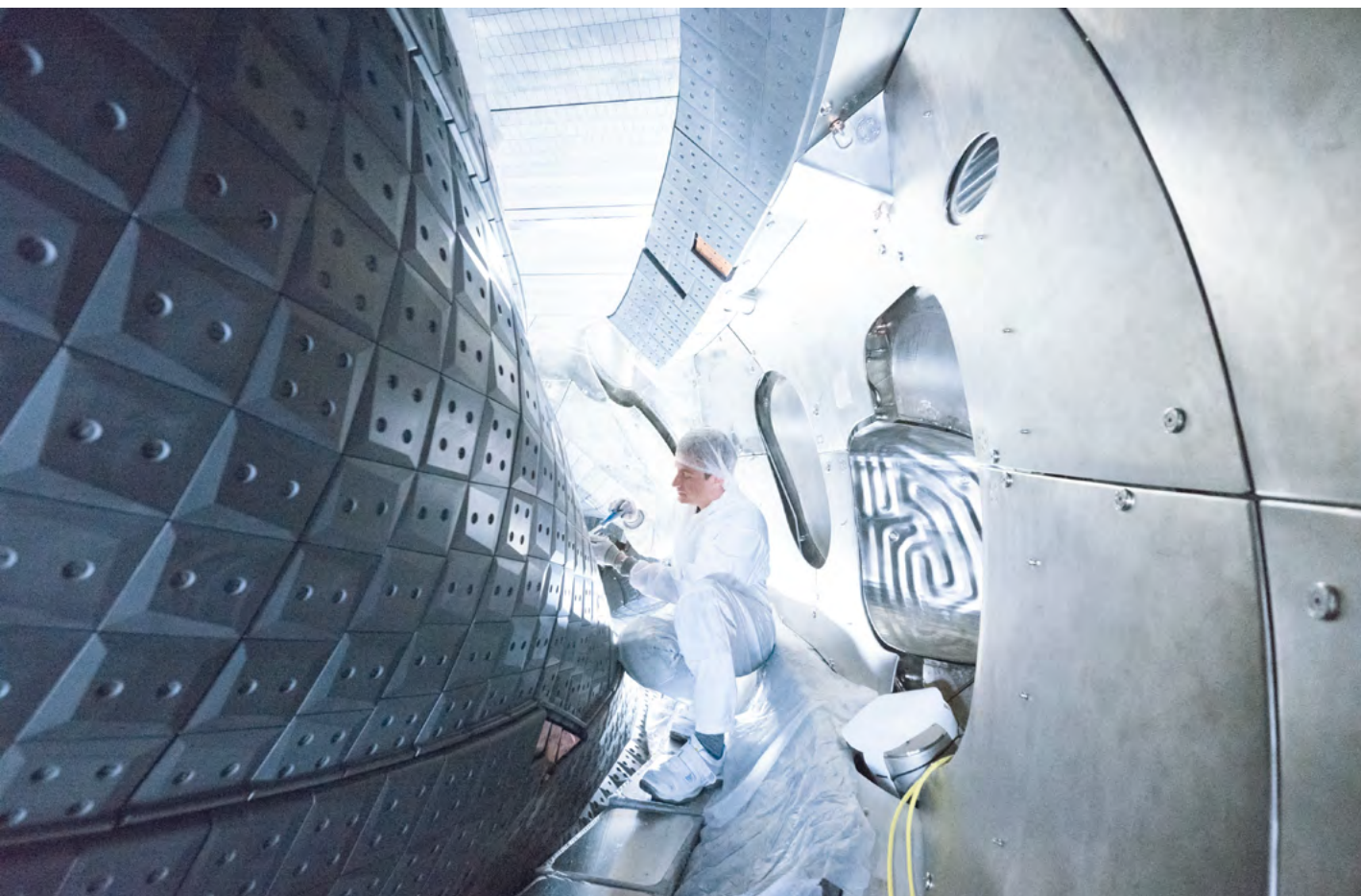
Mounting the graphite tiles in the plasma vessel of the so-called stellarator experiment Wendelstein 7-X at the Max Planck Institute for Plasma Physics in Greifswald.
